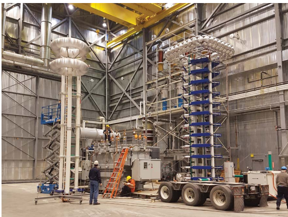
Lightning impulse testing being performed on a 16 MVA power transformer.
